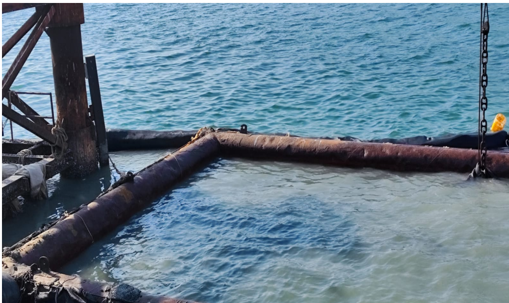
Fig. 3 Connections between Two Adjacent Silt Curtains
