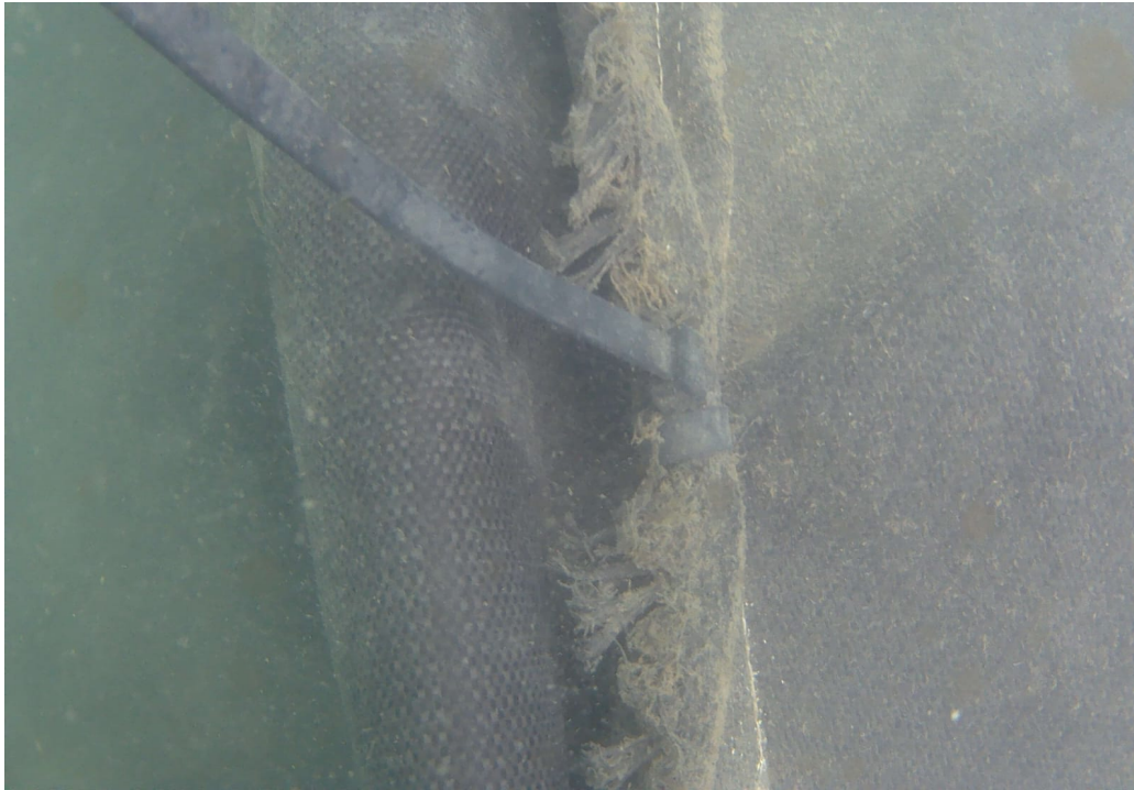
Fig. 10 Connections between Two Adjacent Silt Curtains
