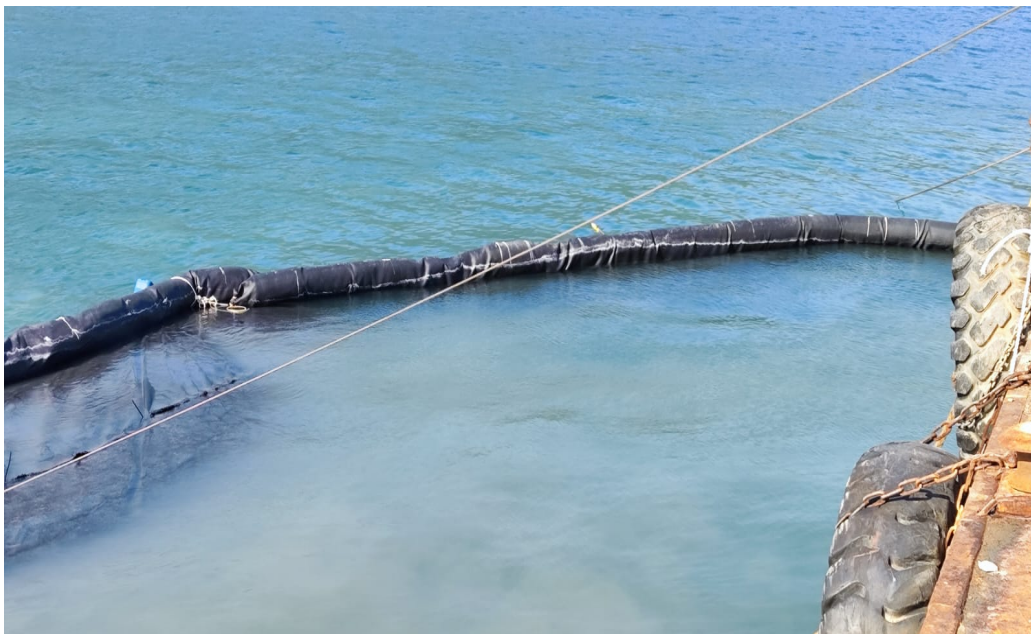
Fig. 5 Connections between Two Adjacent Silt Curtains
