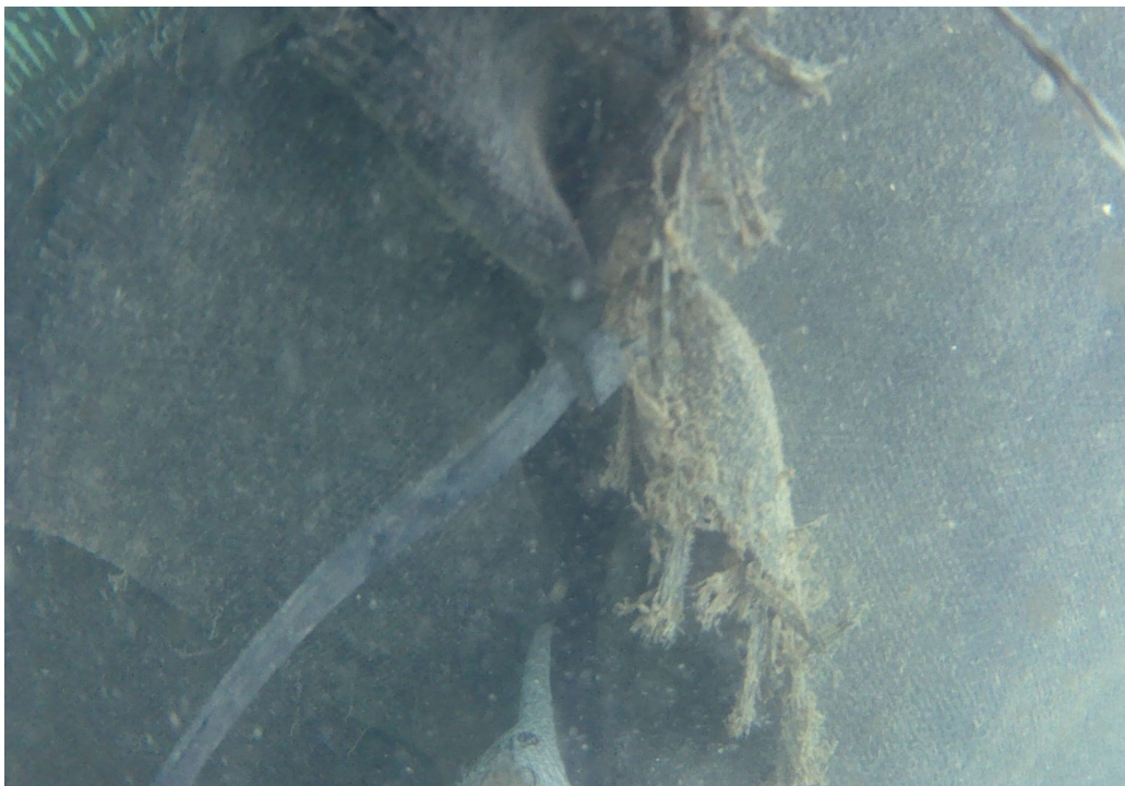
Fig. 9 Connections between Two Adjacent Silt Curtains
