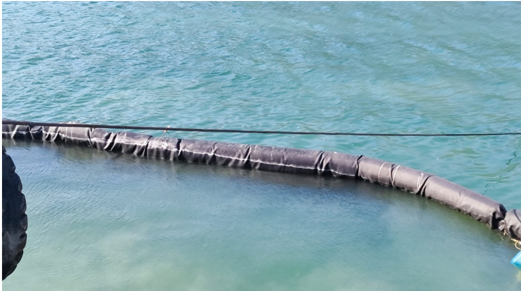
Fig. 2 Connections between Two Adjacent Silt Curtains
