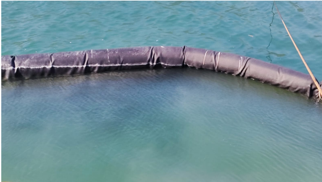
Fig.4 Connections between Two Adjacent Silt Curtains
